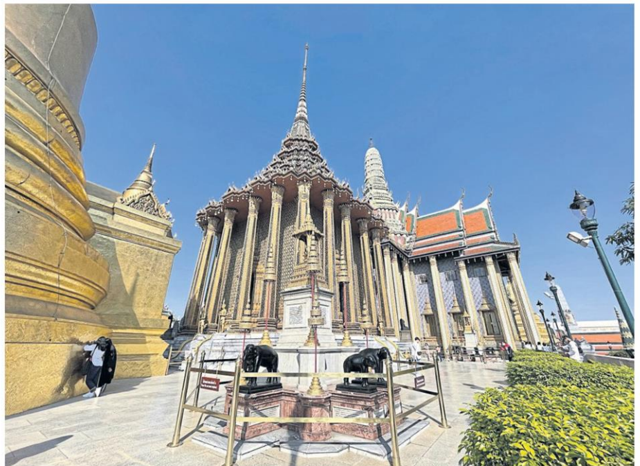
Phra Mondop was constructed during the reign of King Rama I as a library.
